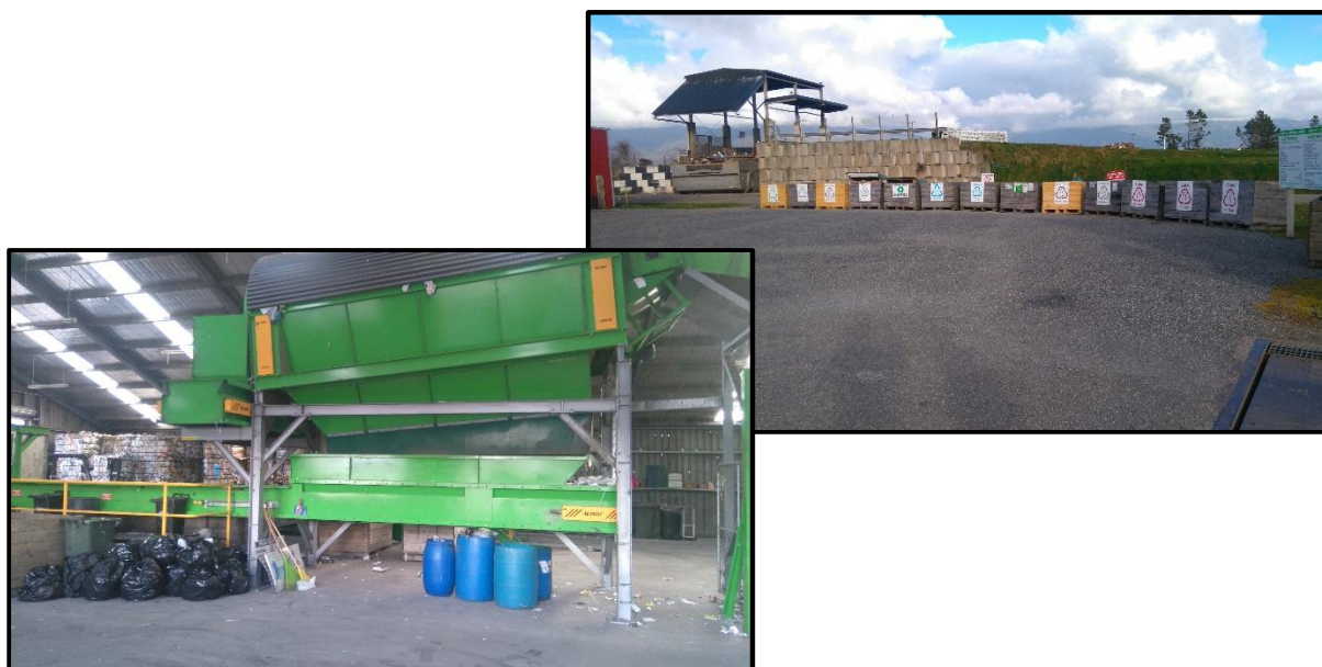
Figure 7: Westport Transfer Station - Drop-off area and MRF
