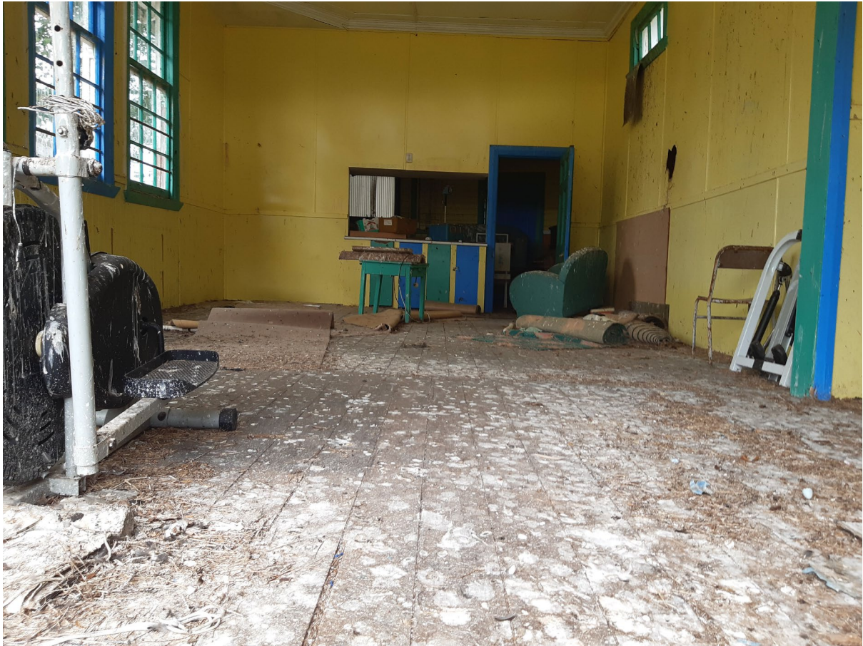
Photo 2: Mawheraiti Hall Interior February 2023
