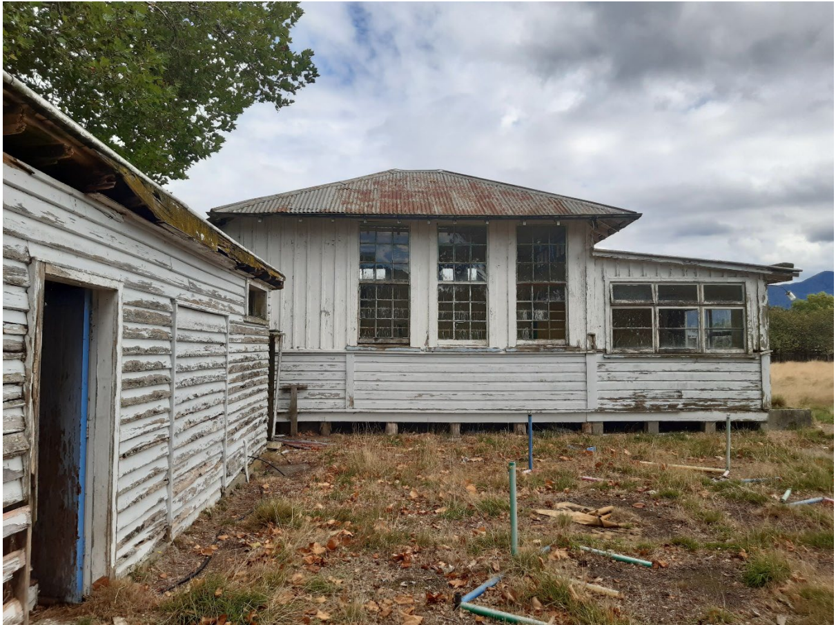
Photo 1. Exterior Mawheraiti Hall February 2023
