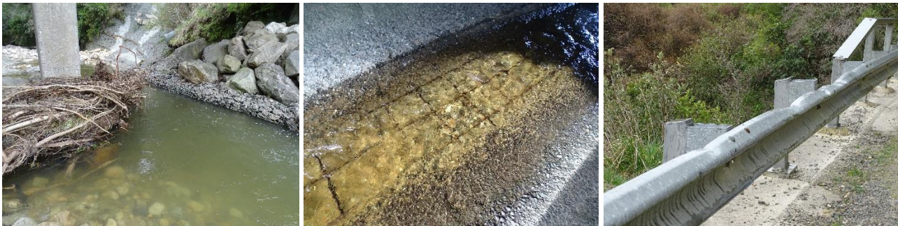
Figure 4: Routine, Structural & Guardrail Maintenance
