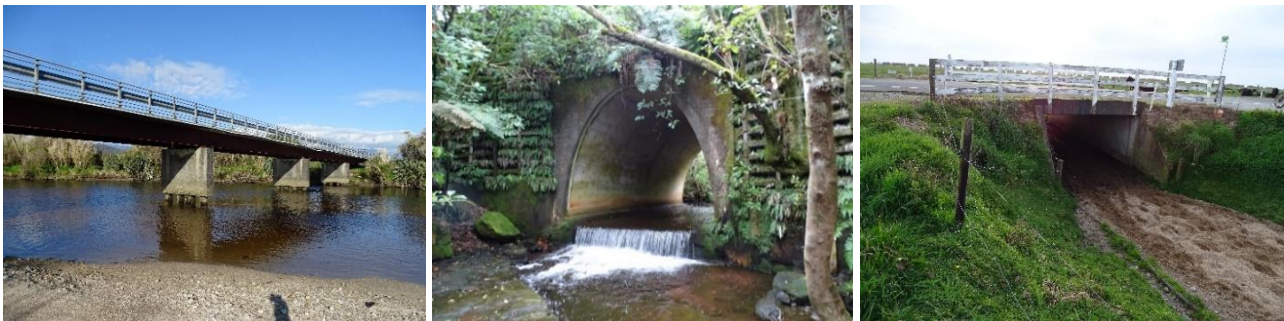
Figure 1: BDC Bridges, Major Culverts & Stock Underpasses
