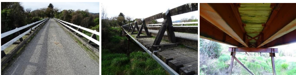
Figure 2: Bridge Descriptive Photographs
