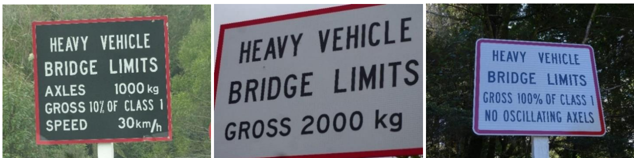
Figure 7: Heavy Vehicle Bridge Limits
