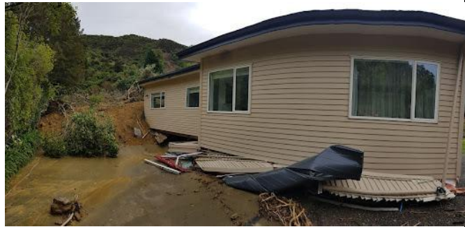
Figure 11. Approximately 2m depth of clay-based landslide debris has pushed this house off its foundation (piles) and moved the building as a complete unit (example from Marlborough).
