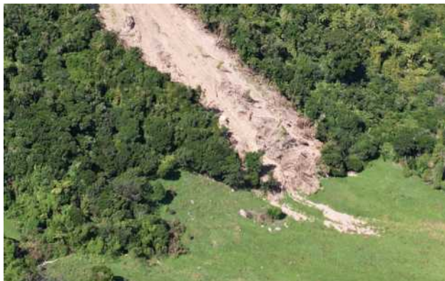
Figure 8. Landslide debris composed
