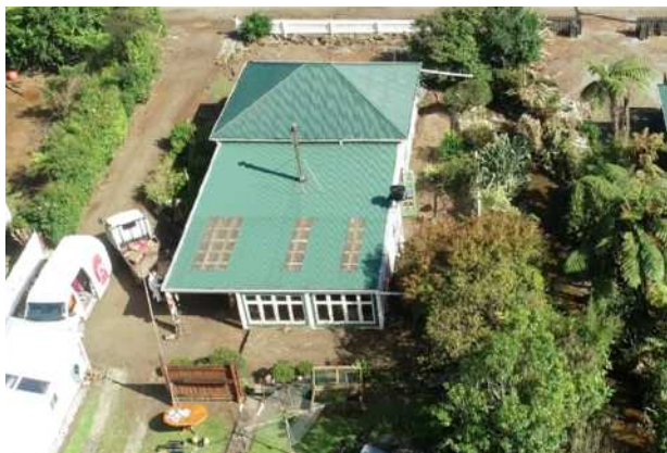
Figure 15. Debris flow deposition around a house in Granity. Approximate depth of inundation is <0.5m. Photo: BDC
